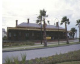
1 railway station complex beach road port melbourne front elevation mar1999
