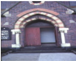
methodist church nicholson street fitzroy entrance aug1980
