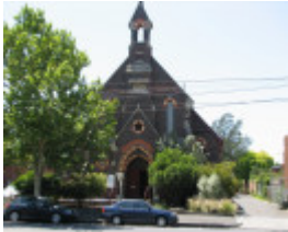
FORMER METHODIST CHURCH SOHE 2008
