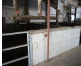
MILDARA BLASS DISTILLERY SOHE 2008
