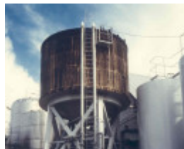
h01099 mildara blass distillery merbein water tank
