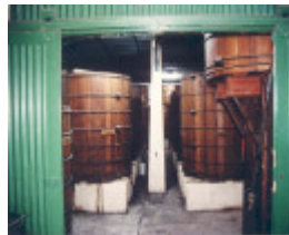
h01099 mildara blass distillery merbein brandy store
