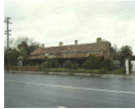
1 iron cottage brunswick road brunswick housing row 1992
