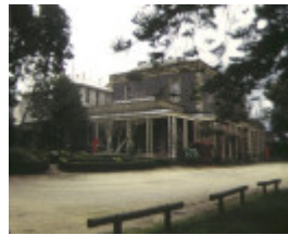
1 morongo bell post hill additions to south side of house
