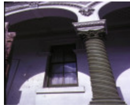
residence 122 nicholson street fitzroy balcony column detail
