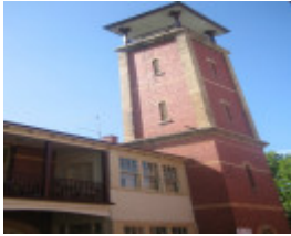
Prahran Volunteer Fire Station_Watchtower_Jan 2008_mz
