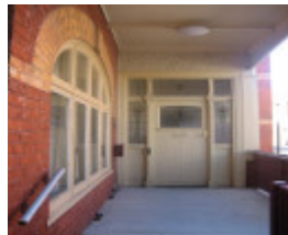
Prahran Volunteer Fire Station_Front Porch_Jan 2008_mz
