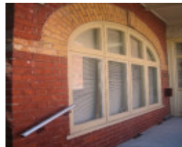
Prahran Volunteer Fire Station_Former Front Door_Jan 2008_mz
