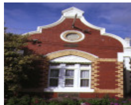
1 coppin avenue 8 coppin avenue front window aug1990
