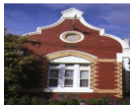
1 coppin avenue 8 coppin avenue front window aug1990
