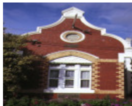
1 coppin avenue 8 coppin avenue front window aug1990
