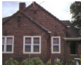
1 coppin avenue & 36 coppin avenue the burdett & mary laycock homes rear view aug1990
