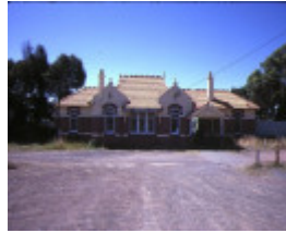
1 wonthaggi railway station front elevation jan1985
