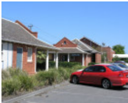
FORMER ROYAL AUSTRALIAN FIELD ARTILLERY BARRACKS SOHE 2008
