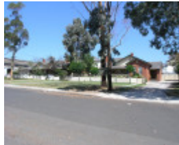
FORMER ROYAL AUSTRALIAN FIELD ARTILLERY BARRACKS SOHE 2008
