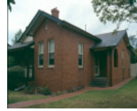
h01098 rafa barracks captain s quarters 2002
