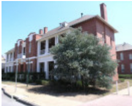
FORMER ROYAL AUSTRALIAN FIELD ARTILLERY BARRACKS SOHE 2008
