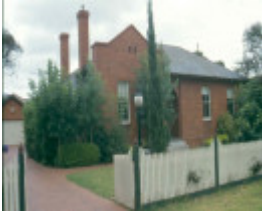
h01098 rafa barracks single men s quarters 2002
