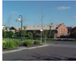
H01098 rafa barracks gun shed 2001pm1
