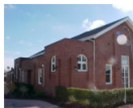
H01098 rafa barracks gymnasium 2001 pm1
