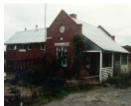
H01098 rafa barracks horse hospital demolished 1995
