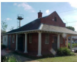
H01098 rafa barracks guard room 2001 pm1
