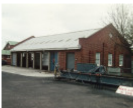
H01098 rafa barracks gun shed 1995
