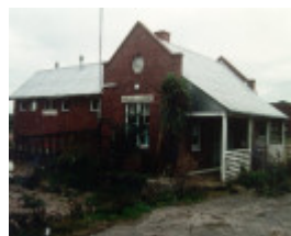
H01098 rafa barracks horse hospital demolished 1995
