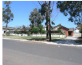
FORMER ROYAL AUSTRALIAN FIELD ARTILLERY BARRACKS SOHE 2008
