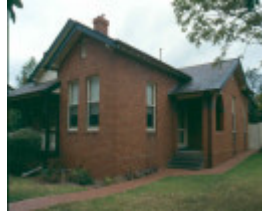
h01098 rafa barracks captain s quarters 2002
