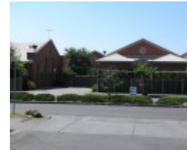
FORMER ROYAL AUSTRALIAN FIELD ARTILLERY BARRACKS SOHE 2008
