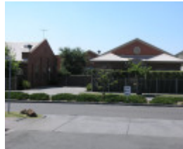
FORMER ROYAL AUSTRALIAN FIELD ARTILLERY BARRACKS SOHE 2008
