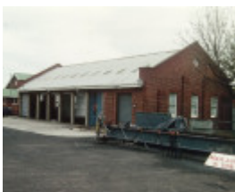
H01098 rafa barracks gun shed 1995
