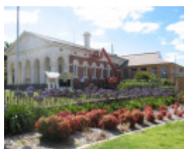
Ararat Shire Hall
