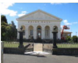
Ararat Shire Hall
