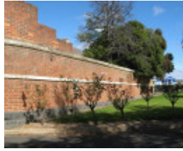
Ararat Civic Precinct brick wall at rear of Shire Hall
