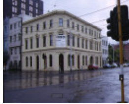
1 former eastern hill hotel victoria parade fitzroy corner view
