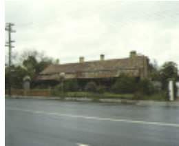
1 iron cottage brunswick road brunswick housing row 1992
