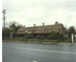
1 iron cottage brunswick road brunswick housing row 1992
