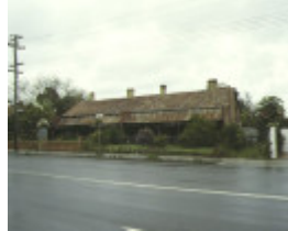
1 iron cottage brunswick road brunswick housing row 1992
