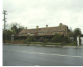
1 iron cottage brunswick road brunswick housing row 1992
