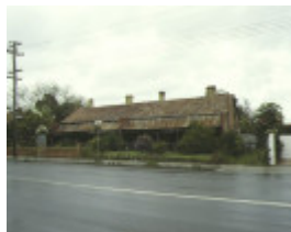
1 iron cottage brunswick road brunswick housing row 1992
