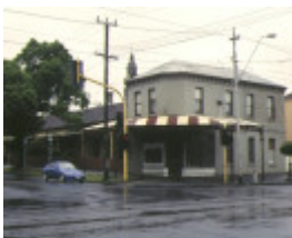
1 park street/emerald hill estate south melbourne 292 park street corner view nov1995
