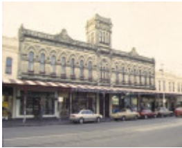
1 park street/1 emerald hill estate south melbourne 256- 264 park street front facade oct1995
