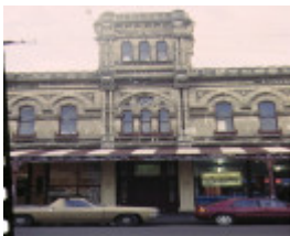
1 park street/emerald hill estate south melbourne 256- 264 park street facade detail oct1995
