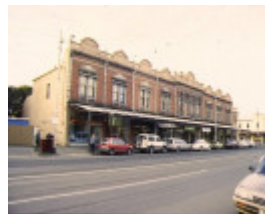
1 park street/emerald hill estate south melbourne 268- 286 park street front view oct1995
