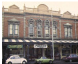
1 park street/emerald hill estate south melbourne 270- 286 park street facade detail oct1995
