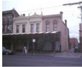
1 park street/emerald hill estate south melbourne 248- 256 park street front view dec1984
