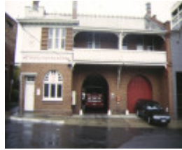
1 hawthorn fire station front view
