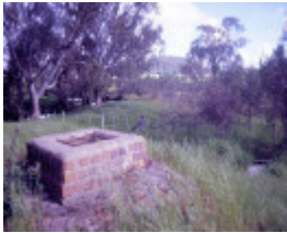
h01330 former thoona dairy and butter factory sargeant street thoona over underground water tank she project 2004
