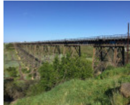
RAIL BRIDGE (ALBION VIADUCT) September 2016
