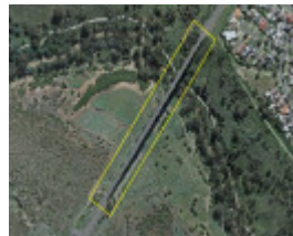
Albion Viaduct Extent Aerial June 2021
