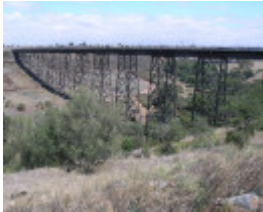
RAIL BRIDGE (ALBION VIADUCT) SOHE 2008
