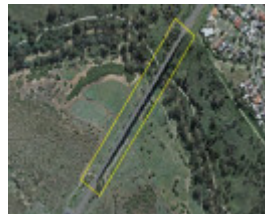
Albion Viaduct Extent Aerial June 2021
