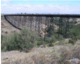
RAIL BRIDGE (ALBION VIADUCT) SOHE 2008
