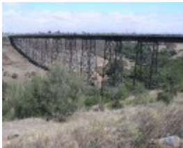
RAIL BRIDGE (ALBION VIADUCT) SOHE 2008
