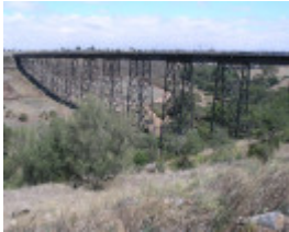
RAIL BRIDGE (ALBION VIADUCT) SOHE 2008
