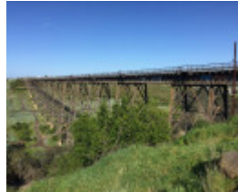
RAIL BRIDGE (ALBION VIADUCT) September 2016
