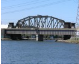
RAIL BRIDGE SOHE 2008
