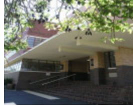
FORMER ESSENDON TECHNICAL SCHOOL SOHE 2008
