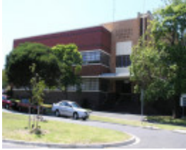
FORMER ESSENDON TECHNICAL SCHOOL SOHE 2008
