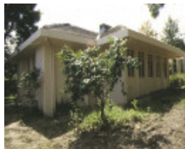
1 murray griffin house heidelberg side view dec1996
