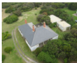
Head keeper's quarters from tower
