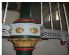
Staircase and column capital
