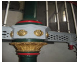
Staircase and column capital
