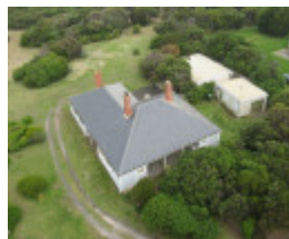
Head keeper's quarters from tower
