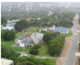
Split Point Lightstation assistant keepers' quarters & stable from tower
