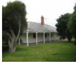
Split Point Lightstation assistants quarters
