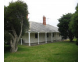
Split Point Lightstation assistants quarters
