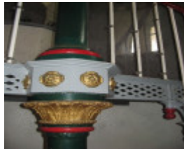
Staircase and column capital
