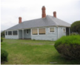
Split Point Lightstation head keeper's quarters
