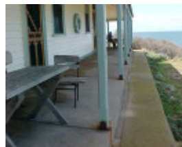
h01983 pt hicks asst qtrs verandah sep03 pm1
