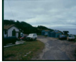
h01983 pt hicks generator shed dec99 pm1
