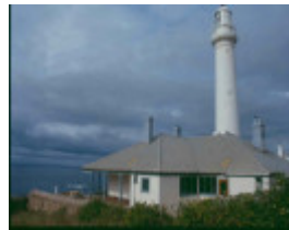
h01983 pt hicks asst keepers qtrs and tower dec99 pm1
