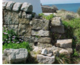
h01983 pt hicks drywall damage3 sep03 pm1
