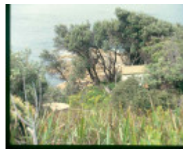
h01983 pt hicks pump house dec99 pm1
