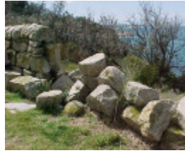
h01983 pt hicks drywall damage1 sep03 pm1
