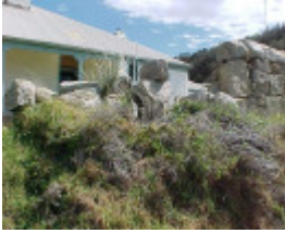
h01983 pt hicks drywall damage2 sep03 pm1
