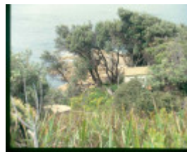
h01983 pt hicks pump house dec99 pm1
