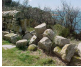
h01983 pt hicks drywall damage1 sep03 pm1
