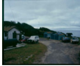
h01983 pt hicks generator shed dec99 pm1
