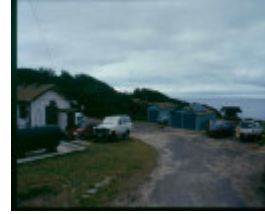
h01983 pt hicks generator shed dec99 pm1
