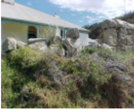
h01983 pt hicks drywall damage2 sep03 pm1
