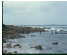
h01983 pt hicks jetty ruins dec99 pm1
