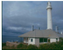
h01983 pt hicks asst keepers qtrs and tower dec99 pm1
