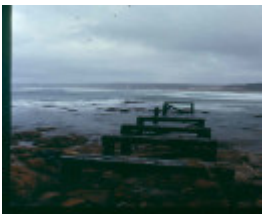
h01983 pt hicks jetty ruins2 dec99 pm1
