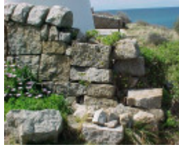
h01983 pt hicks drywall damage3 sep03 pm1
