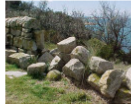
h01983 pt hicks drywall damage1 sep03 pm1
