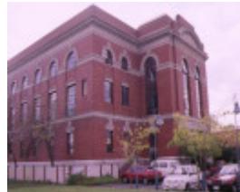
1 former north fitzroy electric railway substation brunswick street north fitzroy side elevation jun1995
