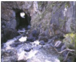
1 blow holes diversion tunnel hepburn tunnel view
