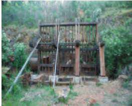
WALLABY MINE GOLD BATTERY SITE SOHE 2008
