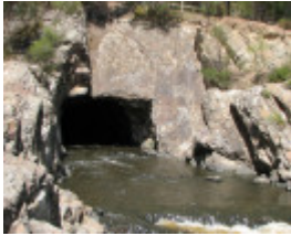
POUND BEND GOLD DIVERSION TUNNEL SOHE 2008
