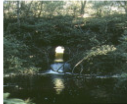
1 houghtons flat gold diversion tunnel nicholson river deptford front view
