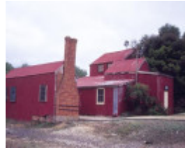
h01264 1 maldon state battery adair street maldon chimney assay room she project 2003
