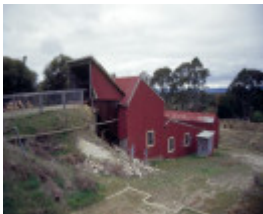
h01264 maldon state battery adair street maldon battery building she project 2003
