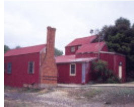
h01264 1 maldon state battery adair street maldon chimney assay room she project 2003
