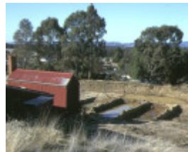
h01264 maldon state battery adair street maldon pits jul1994
