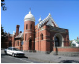
FORMER FLEMINGTON COURT HOUSE SOHE 2008
