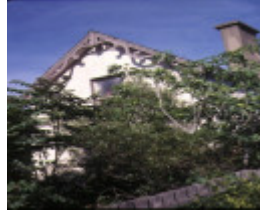
1 residence 39 nicholson street abbotsford view of gable
