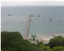
Jetty & surrounds - view from hill, Jan 2008
