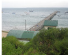
Jetty & shed - view from hill, Jan 2008
