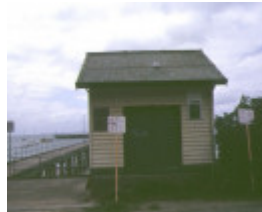
former jetty cargo shed flinders foreshore flinders entrance view
