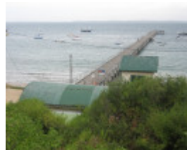
Jetty & shed - view from hill, Jan 2008
