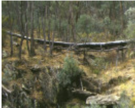
1 red hill hydraulic gold sluicing site castlemaine pipe line side view
