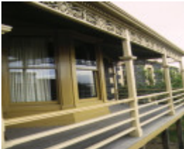
henderson house footscray verandah detail
