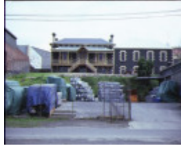
1 henderson house footscray front view
