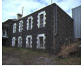
henderson house footscray bluestone building
