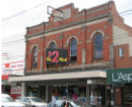
FORMER BATES BUILDING SOHE 2008
