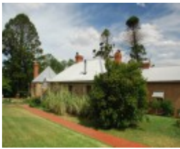
ADELAIDE VALE HOMESTEAD AND OUTBUILDINGS SOHE 2008
