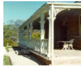
adelaide vale homestead and outbuildings goornong verandah
