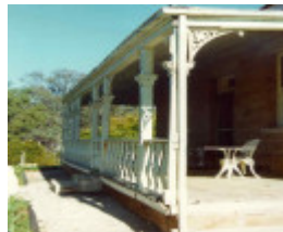
adelaide vale homestead and outbuildings goornong verandah
