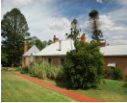
ADELAIDE VALE HOMESTEAD AND OUTBUILDINGS SOHE 2008
