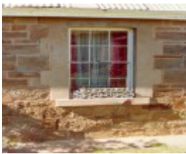
adelaide vale homestead and outbuildings goornong window detail
