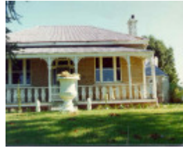
1 adelaide vale homestead and outbuildings goornong front view
