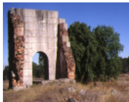
1 duke & timor deep lead gold mine timor pumping engine building rear view mar1998
