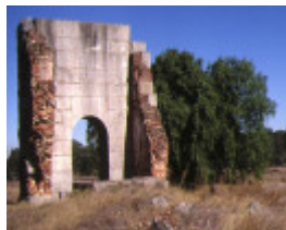
1 duke & timor deep lead gold mine timor pumping engine building rear view mar1998
