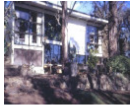
h01313 inge and grahame king house drysdale road warrandyte studios facing north she project 2003
