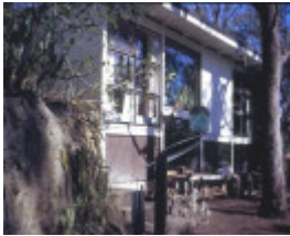
h01313 inge and grahame king house drysdale road warrandyte side view she project 2003
