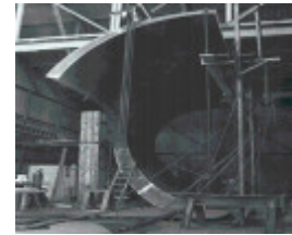
1975-6 Forward Surge under construction .gif
