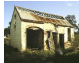
former leaky's residence millers road bacchus marsh stables aug1992
