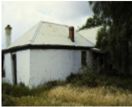
former leaky's residence millers road bacchus marsh rear view
