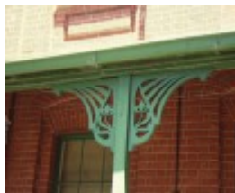
fulham park myrtlebank rd fulham detail verandah
