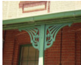
fulham park myrtlebank rd fulham detail verandah
