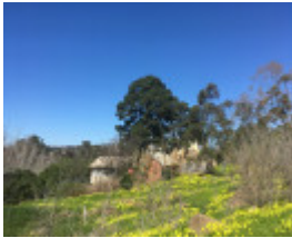
2019 outbuildings and Inn viewed from the north
