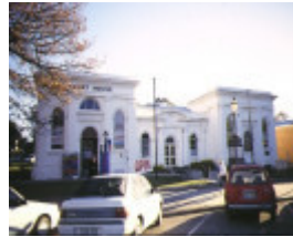
1 former heathcote court house & shire council chambers front view
