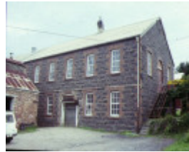
barwon paper mill complex fyansford bluestone building
