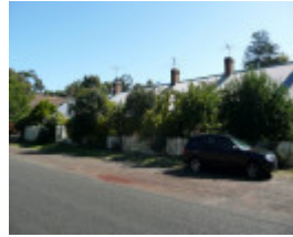
BARWON PAPER MILL COMPLEX SOHE 2008
