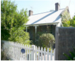
BARWON PAPER MILL COMPLEX SOHE 2008
