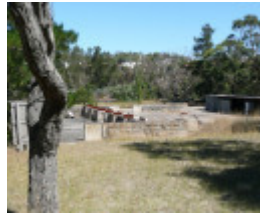
BARWON PAPER MILL COMPLEX SOHE 2008
