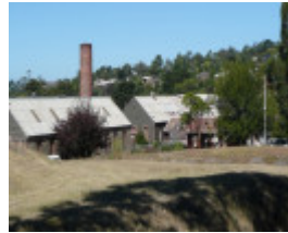
BARWON PAPER MILL COMPLEX SOHE 2008
