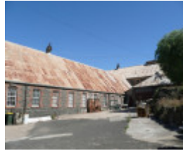
BARWON PAPER MILL COMPLEX SOHE 2008
