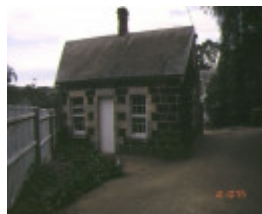
the heights 140 aphrasia street geelong grooms cottage oct1995
