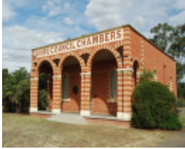
FORMER HUNTLY SHIRE COUNCIL CHAMBERS SOHE 2008
