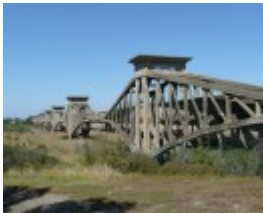
OVOID SEWER AQUEDUCT OVER BARWON RIVER SOHE 2008
