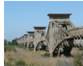
OVOID SEWER AQUEDUCT OVER BARWON RIVER SOHE 2008
