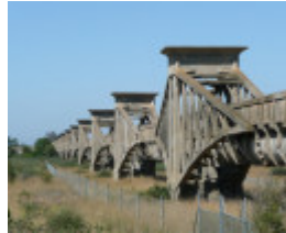
OVOID SEWER AQUEDUCT OVER BARWON RIVER SOHE 2008
