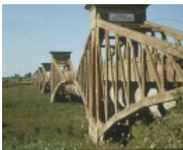
1 barwon river ovoid sewer aqueduct barwon river geelong side view
