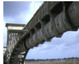
barwon river ovoid sewer aqueduct barwon river geelong view of bottom
