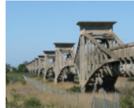
VOID SEWER AQUEDUCT OVER BARWON RIVER SOHE 2008
