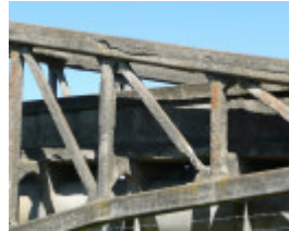
OVOID SEWER AQUEDUCT OVER BARWON RIVER SOHE 2008
