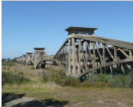
OVOID SEWER AQUEDUCT OVER BARWON RIVER SOHE 2008
