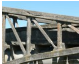
OVOID SEWER AQUEDUCT OVER BARWON RIVER SOHE 2008
