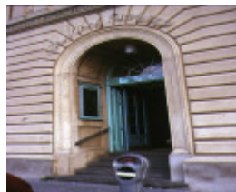
former geelong wool exchange corio street geelong detail of front entrance
