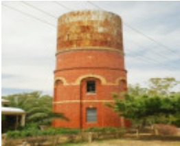
FORMER ELMORE WATER TOWER SOHE 2008
