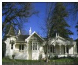
1 corio villa geelong front view
