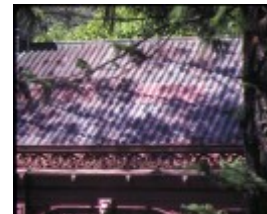
corio villa eastern beach road geelong cast iron roof and lacework
